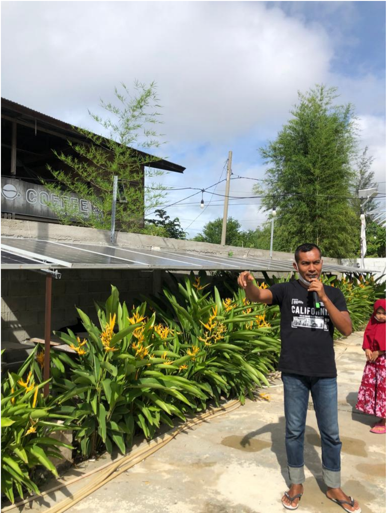
The resource person is explaining directly the process of converting solar energy into electrical energy through the solar panels in the cafe.
